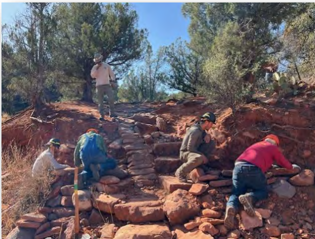
New steps and retaining wall on Old Post
