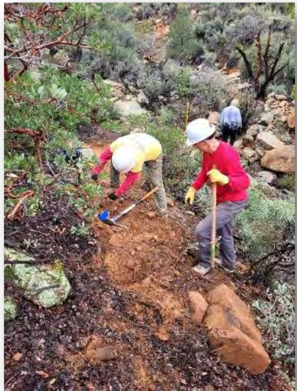
Rock clearing and trail armoring to prevent erosion
